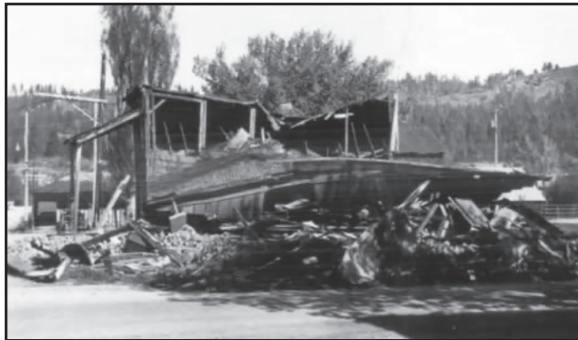
In 1952, the building collapsed due to neglect.
