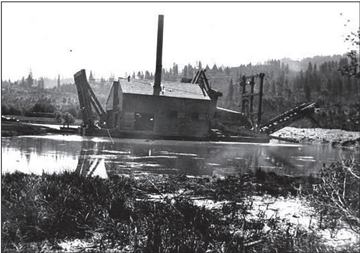
By Skip Myers IDAHO CITY -- Open connected bucketline “Risdon” type dredge operated at Warm Springs near Idaho City, Idaho August 1899. This steam powered dredge was one of the first dredges operated successfully in the Boise Basin. This is near Warm Springs, located about a mile West of Idaho City.
