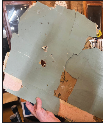
Original paint and wallpaper from inner wall.
