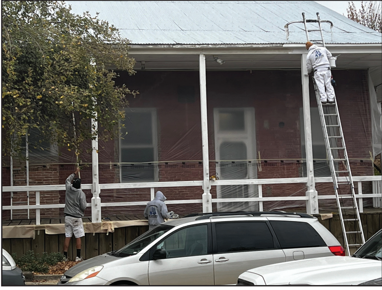
The Boise County Courthouse in Idaho City received a new face-lift the end of October. Painters worked to repaint the outside before the snow arrives, to keep this historical building in pristine condition for the future. Photo by Georgene Thomas
