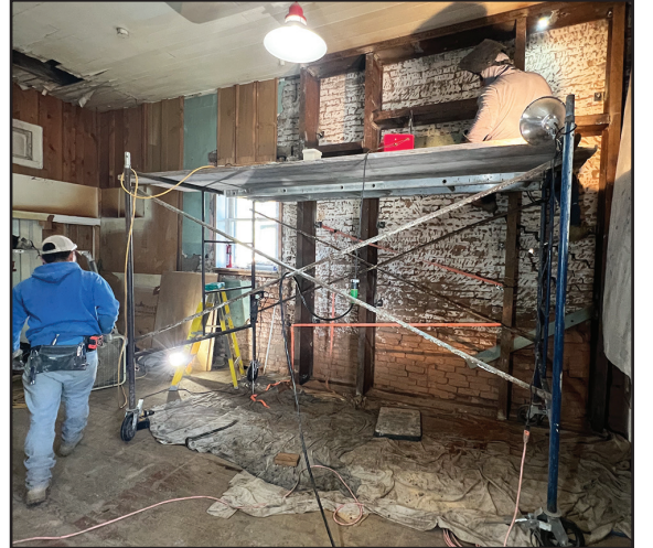
Bracing the wall with I-beams that will double as shelves.
