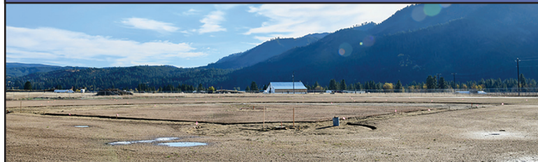
Eight truckloads of sand in place at the new baseball field.
