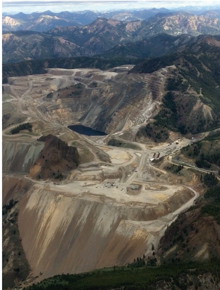
The Thompson Creek Mine is one of the largest molybdenum mines in the U.S. and is located in the Salmon-Challis National Forest. This open pit concept is being considered further down the line for this mineral deposit located north of Idaho City. Photo by Eileen Capson, courtesy of the Idaho Conservation League in 2018.
