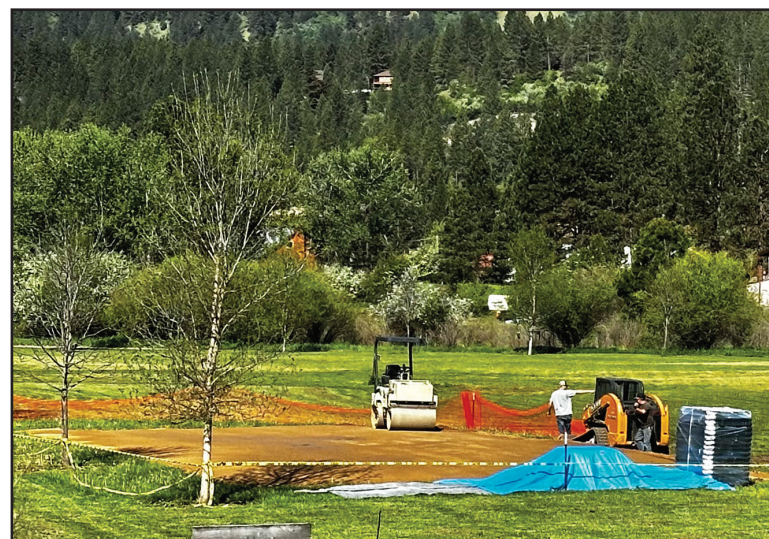
Ground prep raising the "floor" up several feet.
