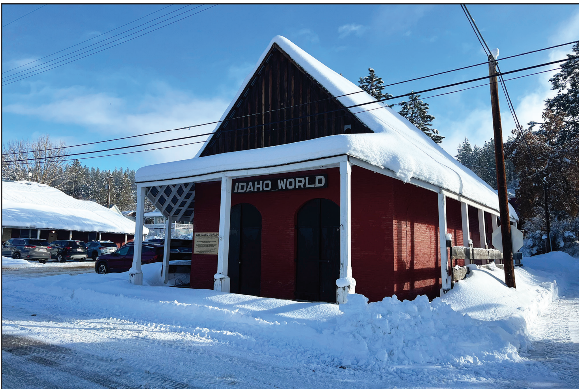
The Idaho World building on Main Street in Idaho City still stands tall after so many winters. This is a registered historical building dating back to the 1800s. A fine silt still filters down through the ceiling, from where it was placed in case of a fire. The thought was that the dirt would extinguish the flames and save the equipment. The building belongs to the Day family and is open to the public in the fall during Idaho City Days. Photo was taken on January 18th, 2024 by Eileen Capson
