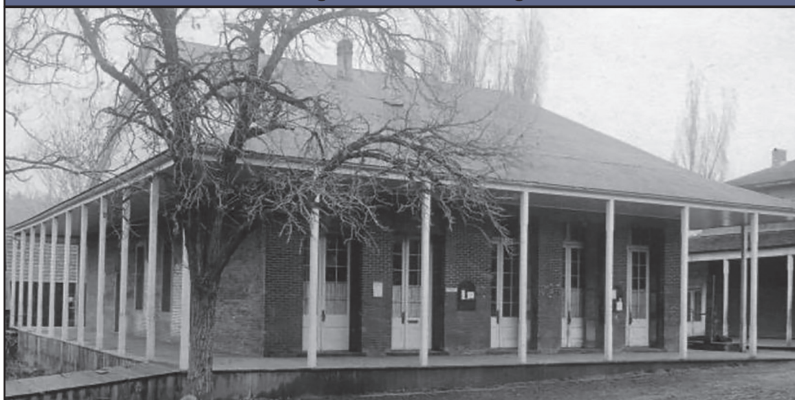
The Boise County Courthouse still stands today on Main Street and is used for court proceedings.
