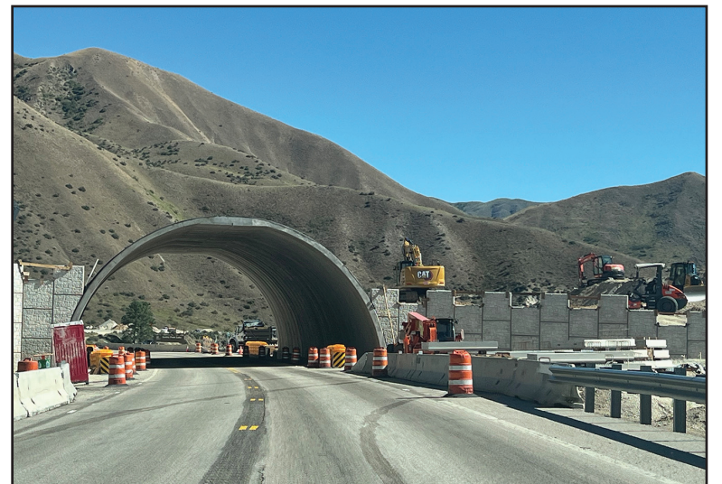
Southbound construction through 25mph zone on August 30.
