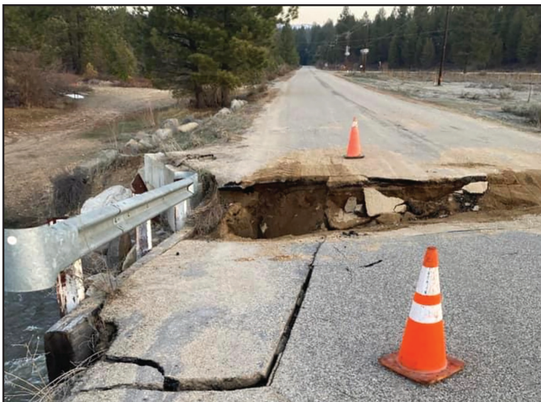
Centerville Road was closed at the Centerville bridge, milepost 4.5, due to a washout on Saturday, April 29th. The Boise County Road Department has been making repairs and it is currently open.
