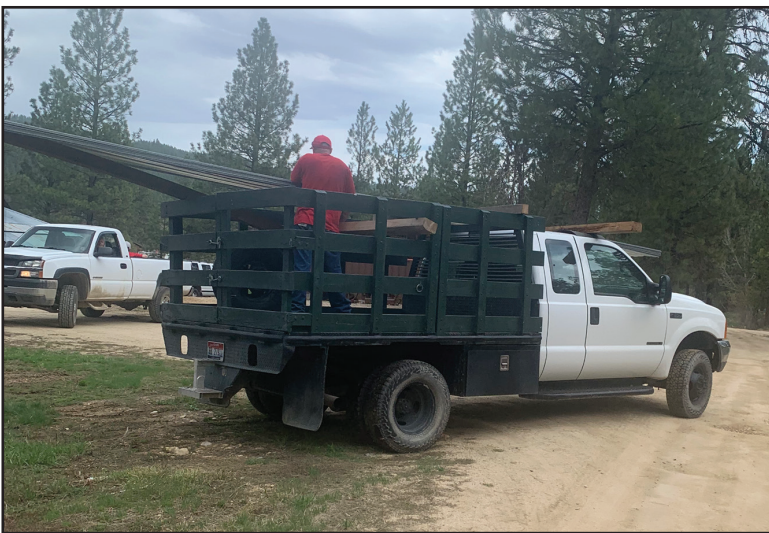
Working with the roofing. Photo by Trudy Jackson
