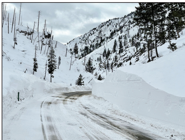
SH-21 Grandjean to Banner Summit after the work done on Friday, March 10th. Provided by the Idaho Department of Transportation
