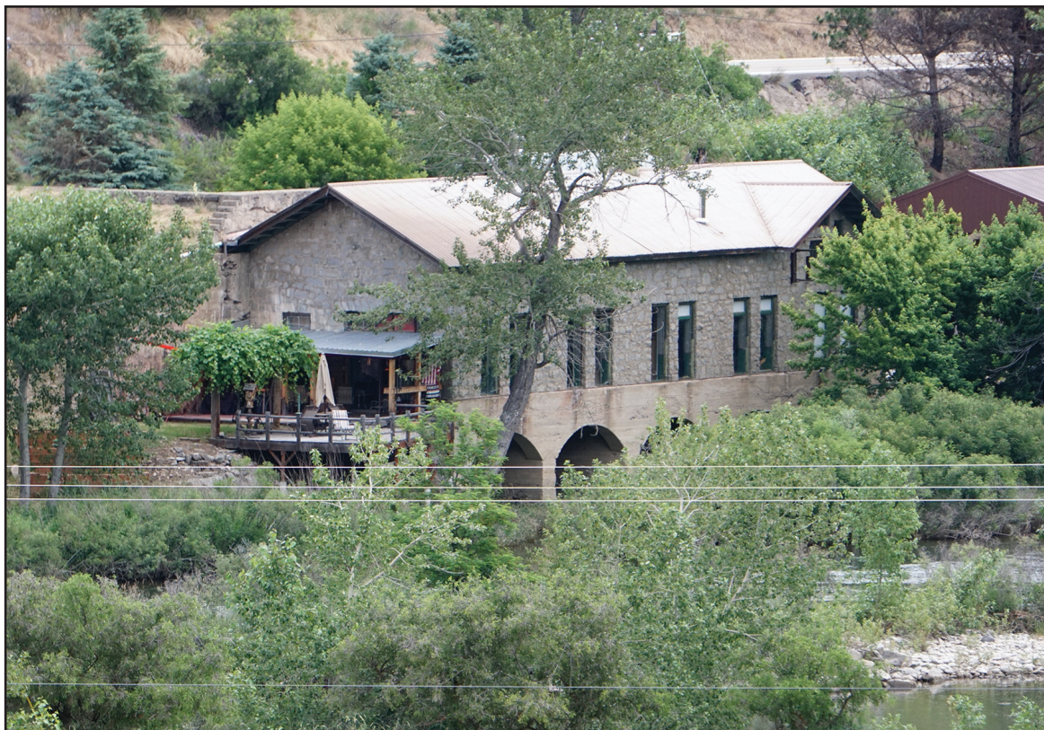
The original Horseshoe Bend power plant still stands in its location along the Payette River. Construction was completed in 1903 and the plant supplied power to street cars and the Pearl Mine.
