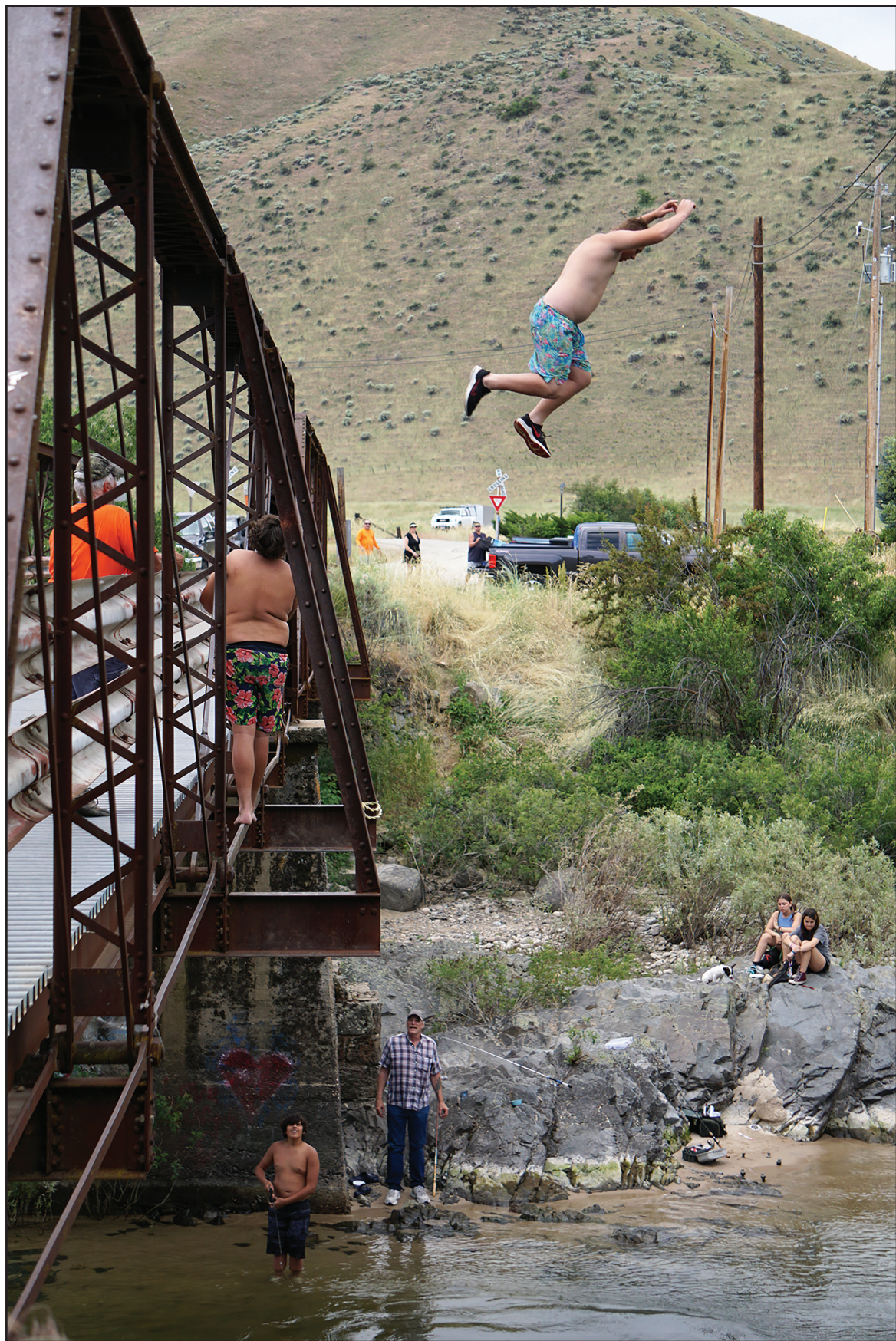
While it may be closed to vehicle traffic, the Boise Road bridge in Horseshoe Bend gets plenty of foot traffic, especially during the warm days of summer when folks want to take a flying leap of faith into the Payette River below. Photo by Tracy Koslosky
