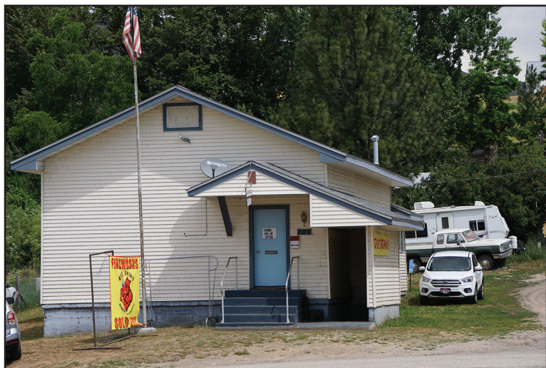
The American Legion Hall was once the Horseshoe Bend Bank Building. Originally a two story structure, the upper portion was destroyed by fire and consequently removed. The bank's safe still resides in the basement.
