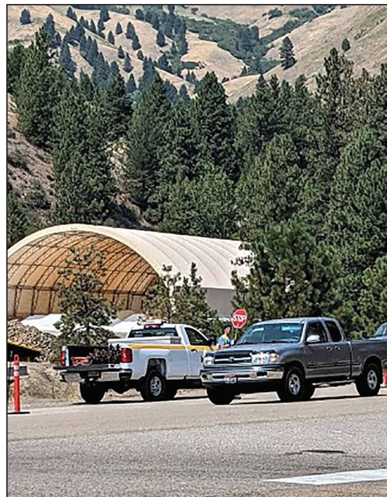
An Idaho Transportation Department flagger directs traffic on Highway 55.
