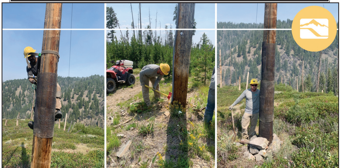
Preventing fire damage and working to keep the power on.
