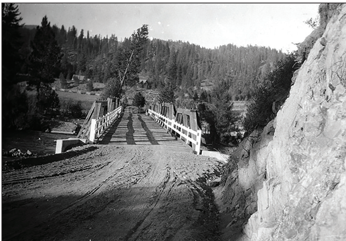
Completed truss bridge
