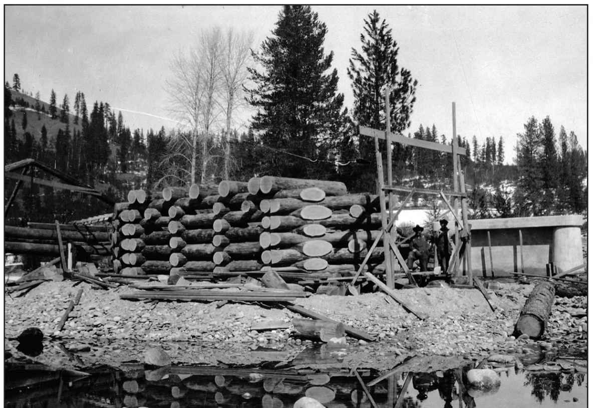
Construction of timber crib center pier.
