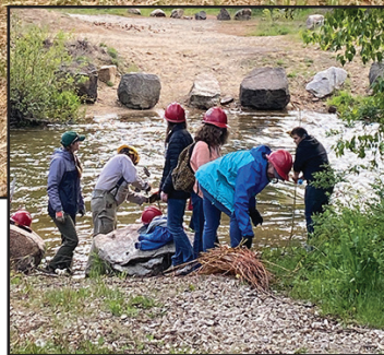
Trimming willow at an angle for better planting and more surface area. Then planting willows, using tools, along the bank of the creek. Photos by Eileen Capson
