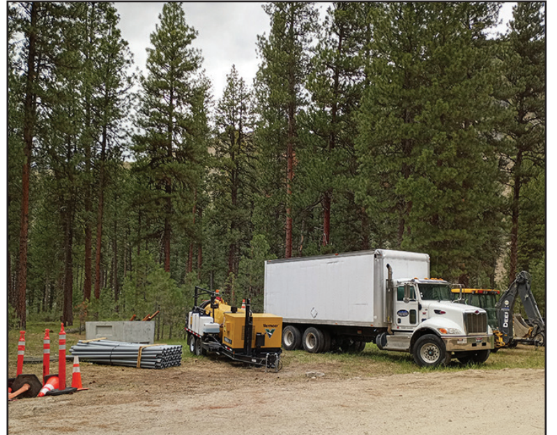
Utility work is set to begin.
