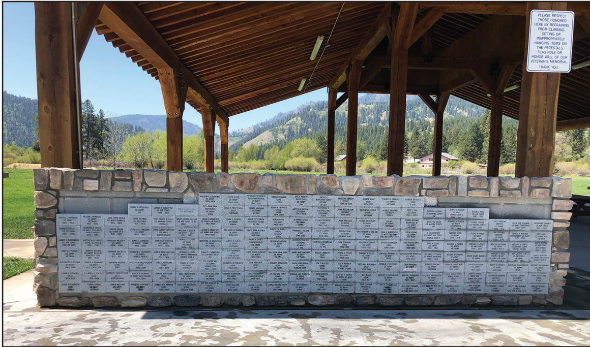
The work was provided by Rose Masonry.
