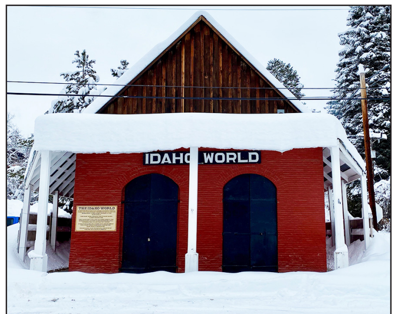
The historic Idaho World building in Idaho City where the newspaper was once printed. This building is on the National Register of Historic Buildings of America. Photo by Eileen Capson
