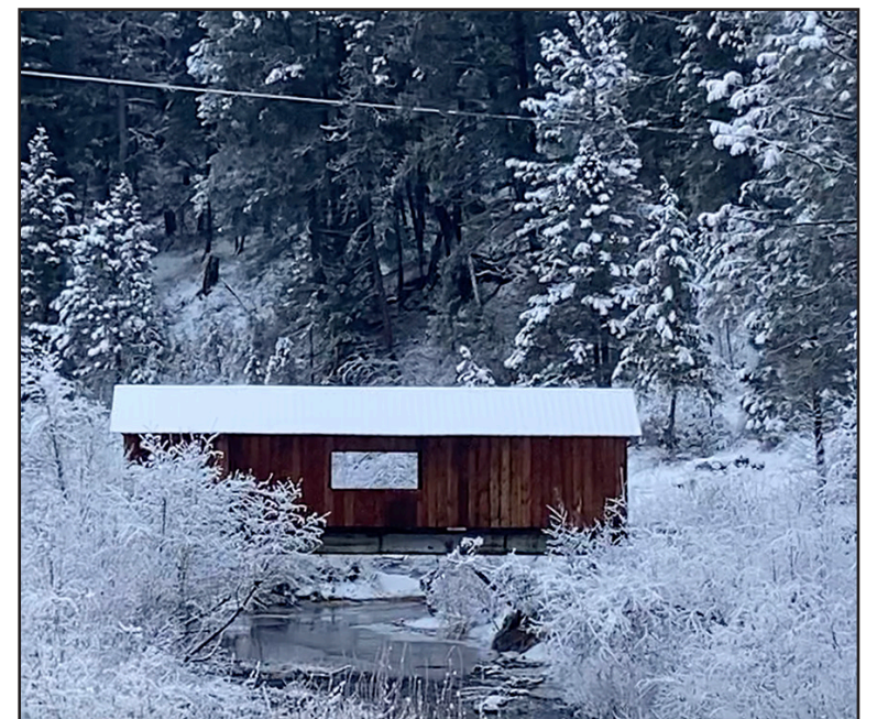
According to the landowner, he has been told that this is the only covered bridge in Idaho. It's located along Hwy. 21. Photo by E. Capson
