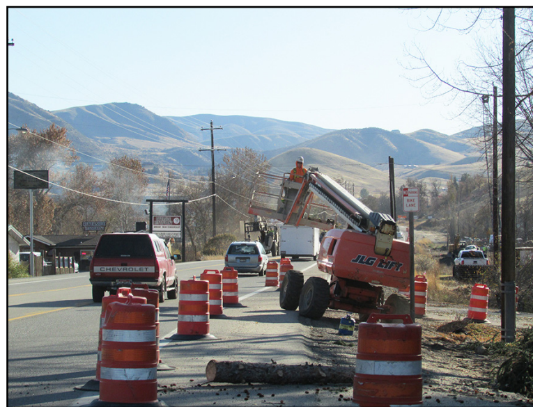
New bridge construction begins in Horseshoe Bend.
