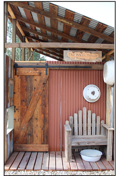
The Wash House - The only coin operated showers from Lowman to Boise! Photo by Eileen Capson
