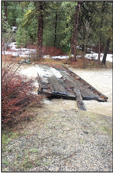
An old bridge located south of Idaho City on Mores Creek. It was a concern that this bridge may take out two others downstream.
