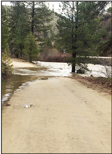
Water on the road near Daggett Creek.
