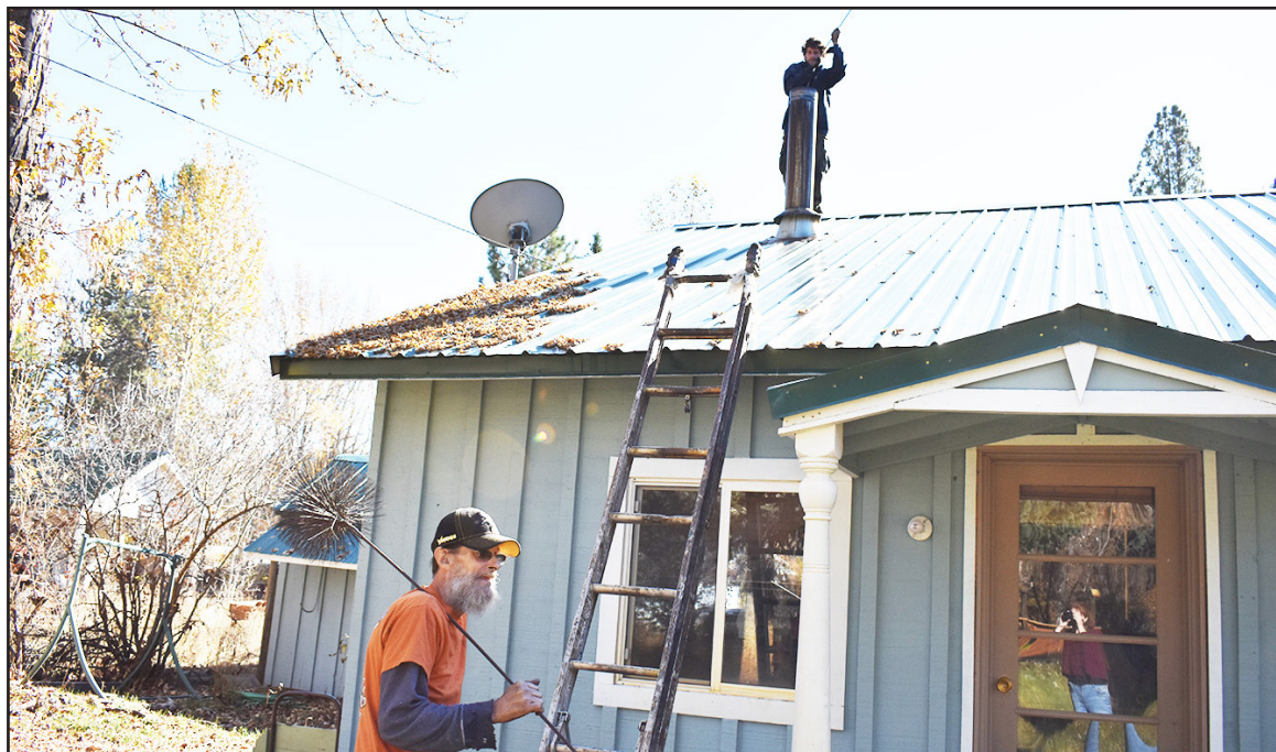
Mark Wedemeyer and his apprentice cleaning a stove pipe in Idaho City. Photo by Eileen Capson
