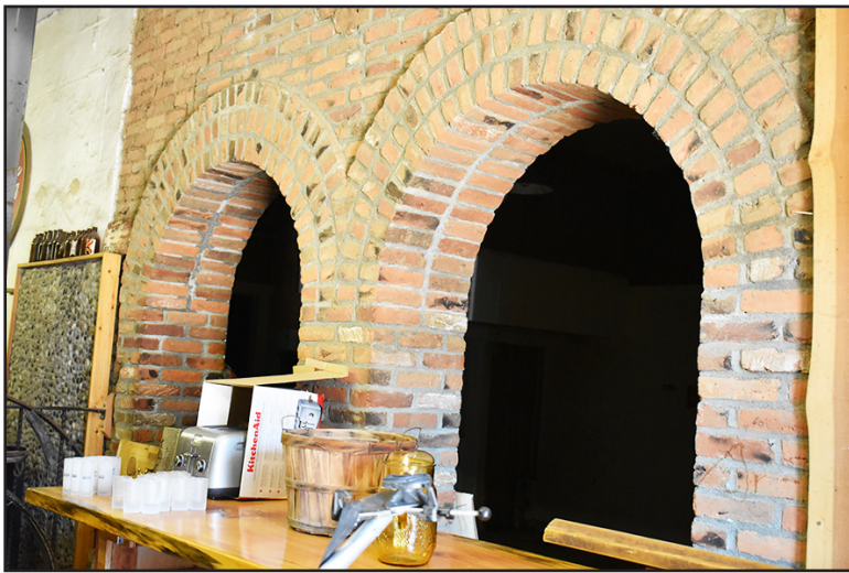
Masonry work at the old Merc. building in Idaho City.
