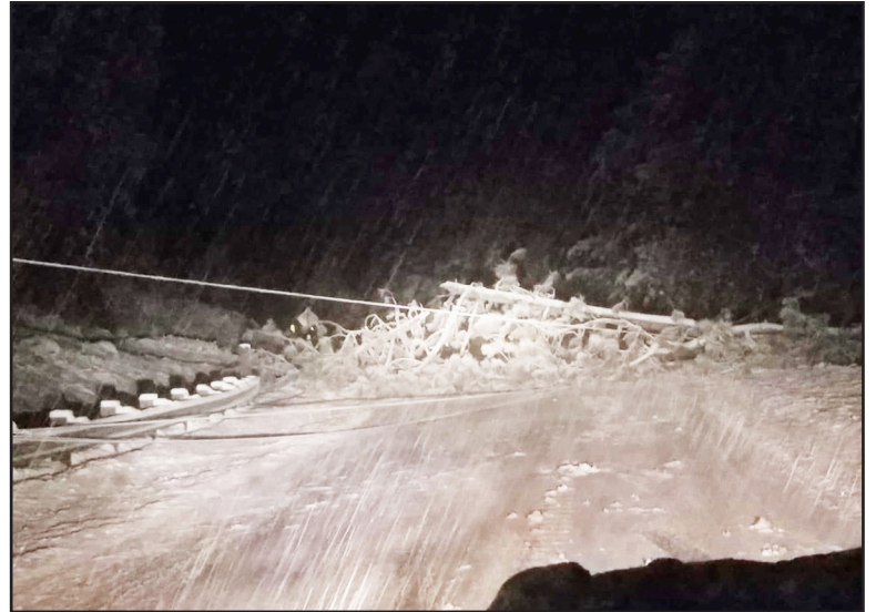
Highway 21 was totally blocked on December 2nd, at 3:30am, when a pine tree fell during a snow storm, falling across the powerlines. Customers in Placerville, Centerville & Idaho City were without power from 2am to 8pm on Sunday.
