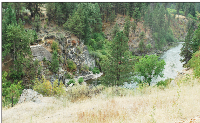
Wharton Dam/ Power House Photos by Jerry Branson
