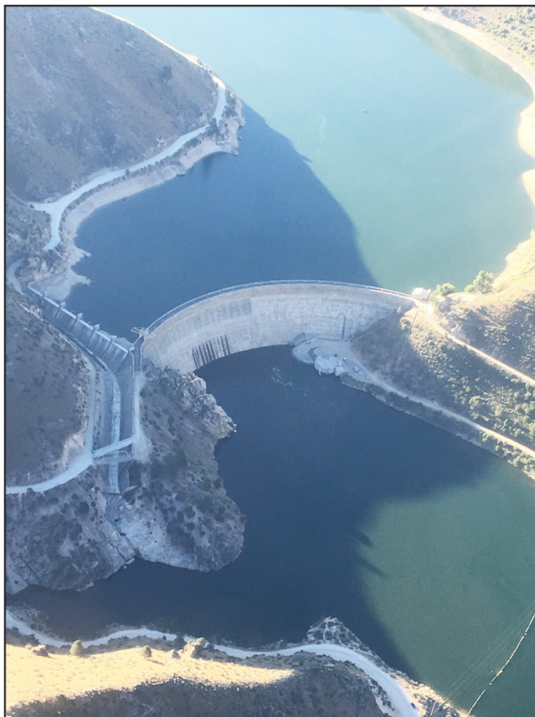
An aerial view of the Arrowrock Dam, which was completed in 1915. It borders Elmore and Boise County. The arch dam measures 225 feet at the base and is 15 feet thick at the top. It is also 350 ft. in height and measures 1,150 ft. in length. Arrowrock was the largest dam, prior to the Hoover Dam, built in 1936. Photo by Eileen Capson
