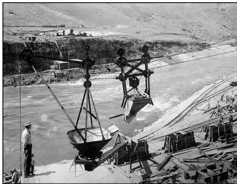
Cement was conveyed to the dam on May 22, 1912. Photo courtesy of the Idaho State Historical Society (ISHS)
