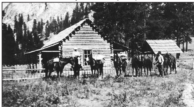
The log cabin of Grandjean, at Grandjean, was done in 1910. John Jackson and Andy Phelps whip sawed the lumber there in late September, 1910. Courtesy of Idaho State Historical Society
