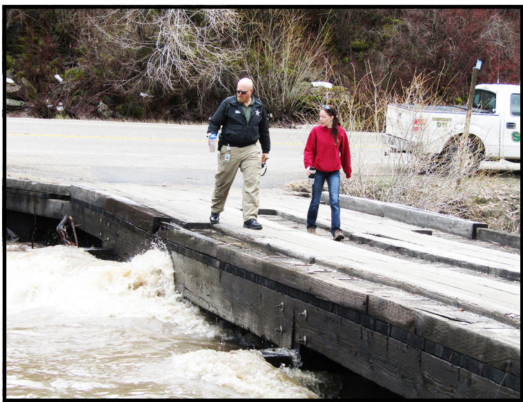
Sheriff Jim Kaczmarek and Camille Wassom, with the Robie Creek Volunteer Fire Dept., kept close tabs on the flooding and threat of debris (aka - trees) from taking out Hummingbird Lane's access bridge.
