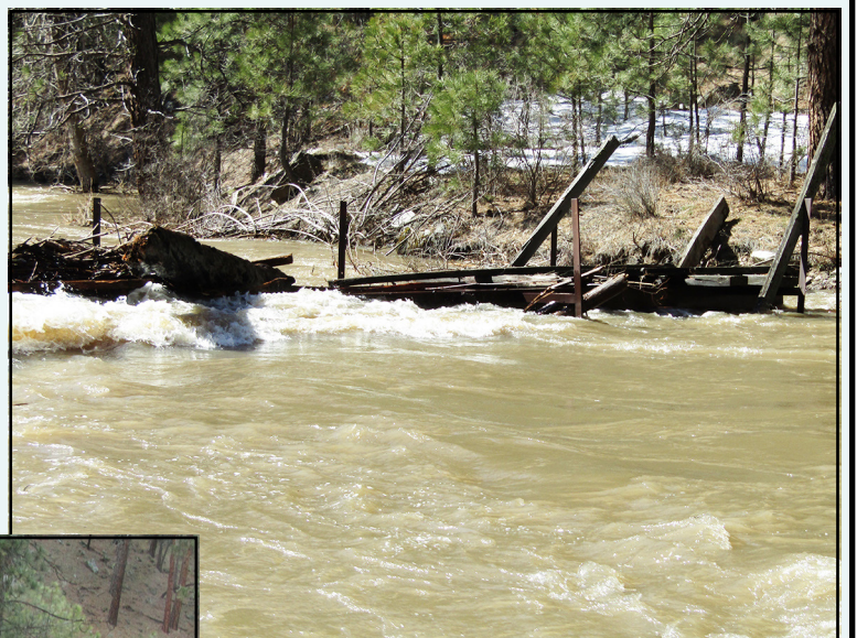
The water level had risen and continued to rise, causing structural damage to Miner Mike's Bridge.
