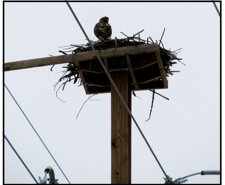
A young osprey returns to its nest. These birds have increasingly chosen to nest on powerpoles. Idaho Power asks the public to notify them, should there be a need for a platform. Otherwise, the nesting materials may fall onto the lines and cause an outage.
