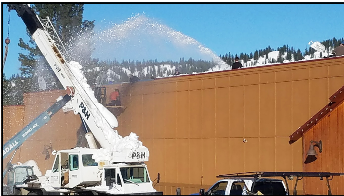
A large snow blower on the roof helped to get an estimated 300 tons of snow off the roof of the Garden Valley Market. A snow conveyor was then used with a crane, to help get the snow removal project done. The weight of the snow was compromising the roof of the Garden Valley Market. Photo by Janet Juroch
