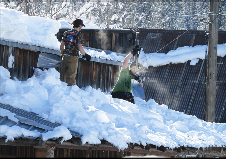
Removing the snow from the roof of a historic building on Main Street in Idaho City. With the temperatures hovering below zero, and staying in the mid-20s during the day, the snow has not shed from the metal roofs. The heavy weight of the snow can be damaging. Photo by Eileen Capson
